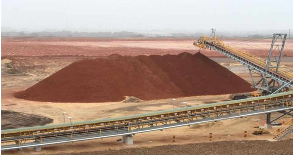
Figure 1. Red mud dry stack facility in Western Australia (Diemme Filtration installation)
